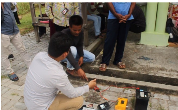
Gambar 10. Pelatihan Pemasangan Power Charge Station
