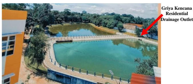
Figure 1. Unila Retention Pond (Embung Rusunawa) [4]
