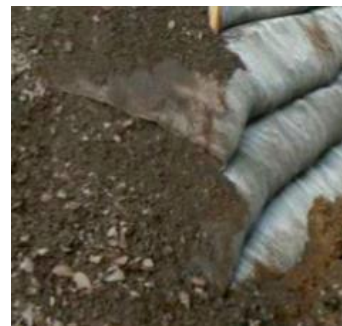
Figure 3. Embankment with insertion of geosynthetics
