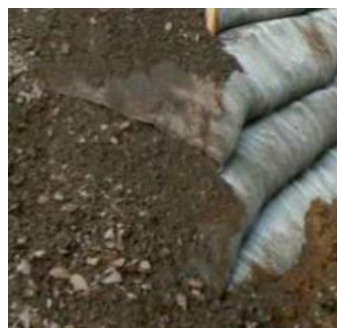
Figure 3. Embankment with insertion of geosynthetics
