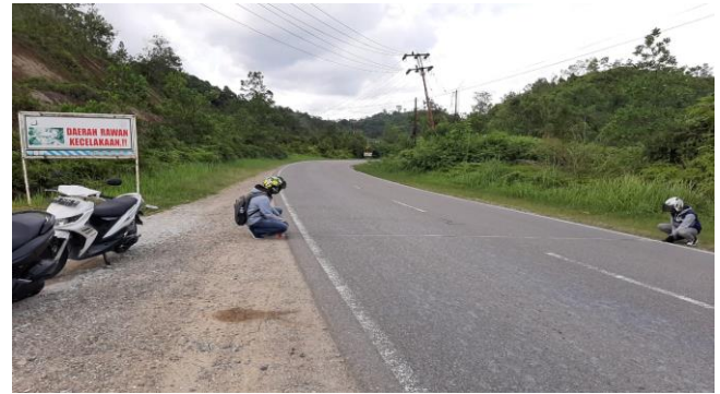
Figure 5. The pavement road of potential traffic accident in Km 92 Merangin Village
